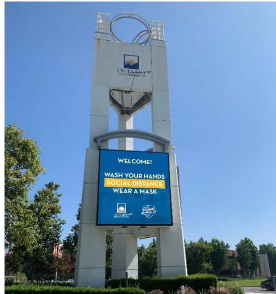
External digital signage, Marquee
